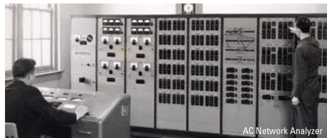
AC Network Analyzer
