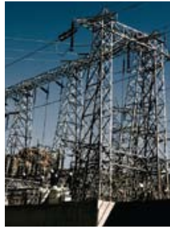
The department plans to build a test bed for cyber security of power systems as well as develop a laboratory that allows researchers to recreate a representative distributed power system.
